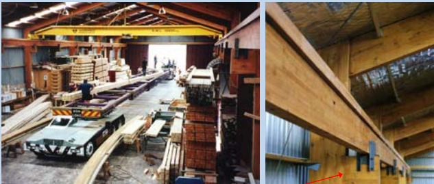
Factory glued corbel for gantry
