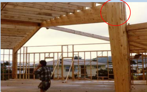
Cross lapped glued joint
