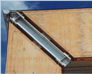
Joint reinforced with a steel profile
