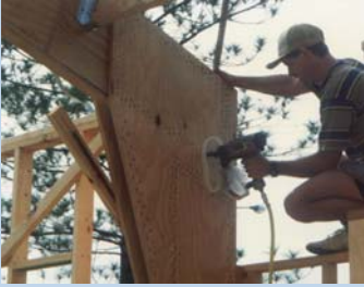
Nailed plywood gussets
