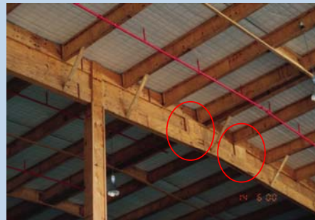
Splicing I-beam rafters
