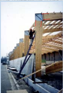
Joints with steel plates and epoxy rods
