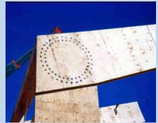
Dowelled cross lapped joint
