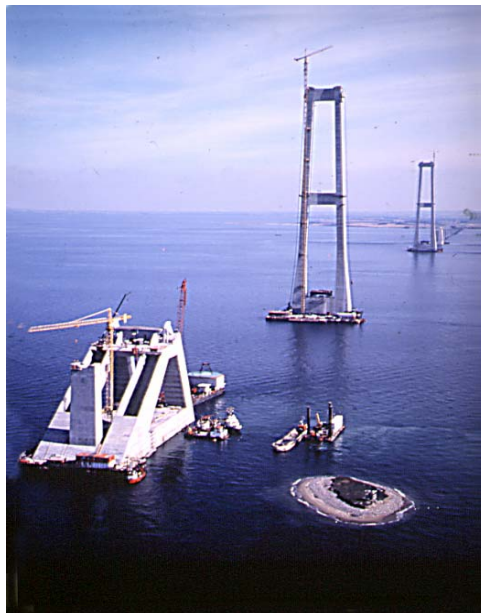
Great Belt Bridge under Construction
