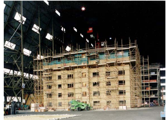
Figure 4: Brick cladding under construction
