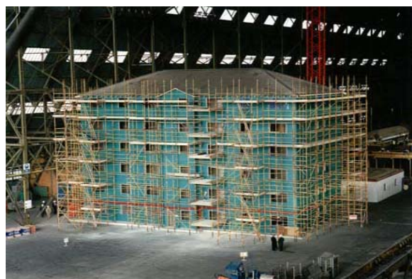
Figure 2: Completed construction stage after 17 days
