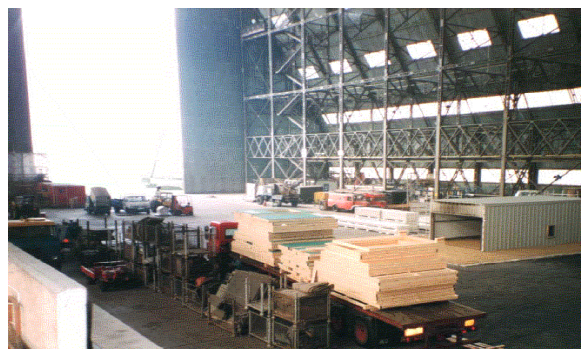
Figure 3: Prefabrication (roof segment on site & wall panels off-site)
