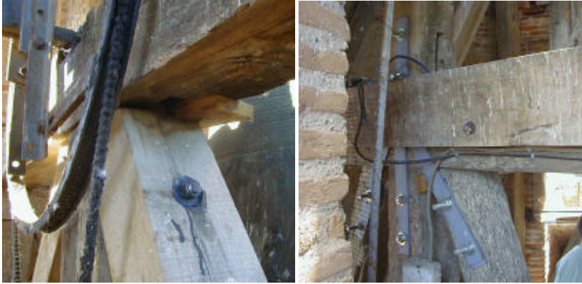
Figure 2 . reinforcement of a joint with a transverse bolt and with bolted steel plates.
